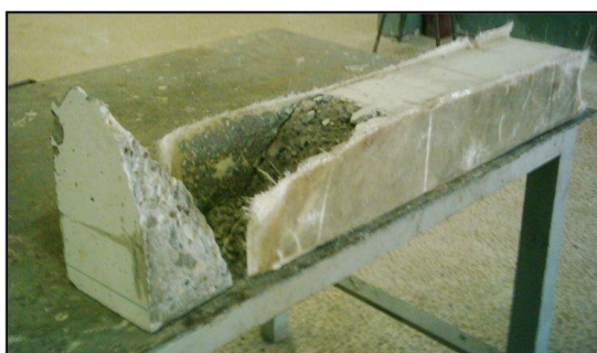
Fig. 3 The failure shape of prisms after debonding GFRP sheets
